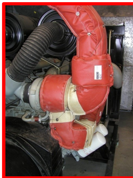
Fabricated cover for turbo-charger and exhaust system piping.
