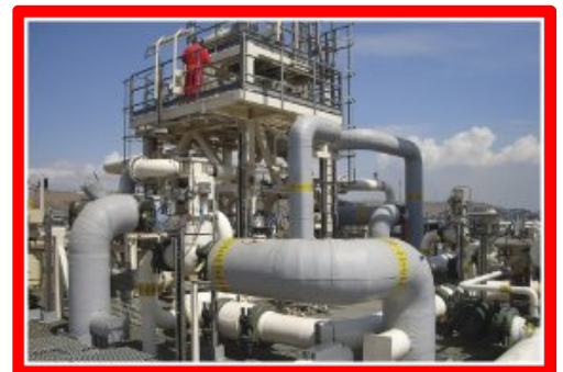
Weatherproof Insulation Page 7-6
